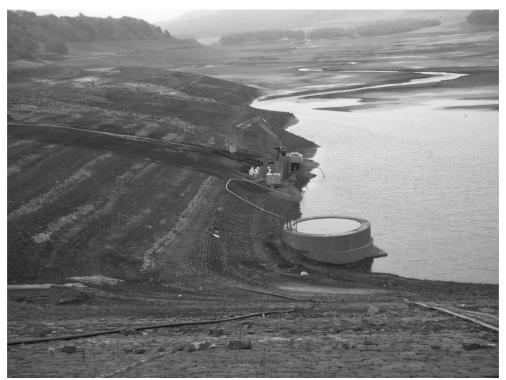
Photo 2 - Excavation at the site of the hole viewed from dam crest. Upstream valve chamber in foreground.
